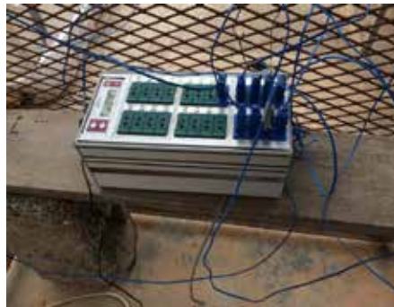
Figure (6). The data acquisition system.
