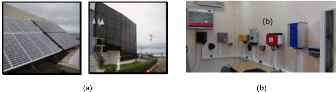
Figure 1 (a) Crystalline silicon PV panels (c-Si, m-Si) on rooftop and thin-film (a-Si, m-Si) on the facade of the UDES building. (b) The control room of the multi-technology PV power plant is connected to the UDES grid.
