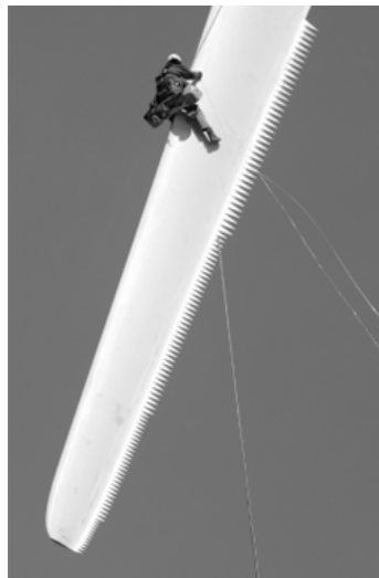
Figure 3. Climber removing trips of the trailing edge serrations mounted on wind turbines blades [55].
