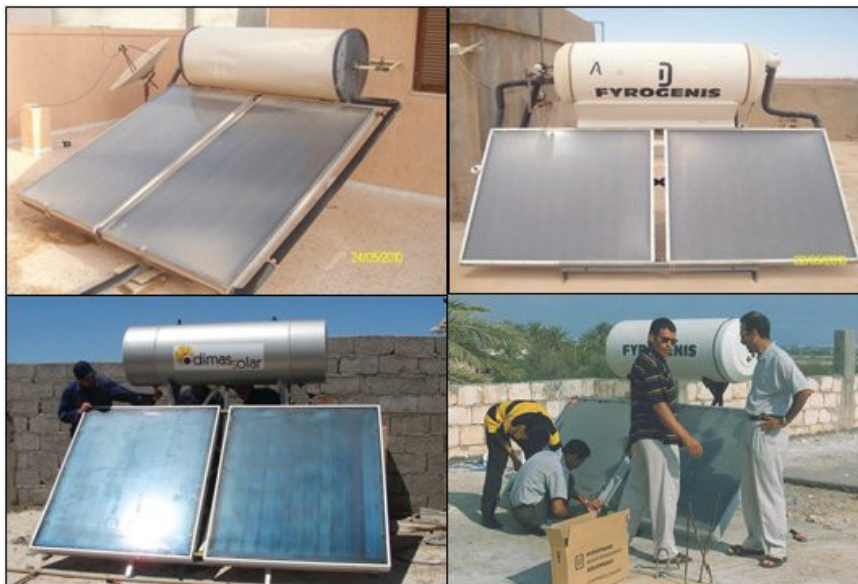
Figure (13). Solar water heaters installation by CSERS
