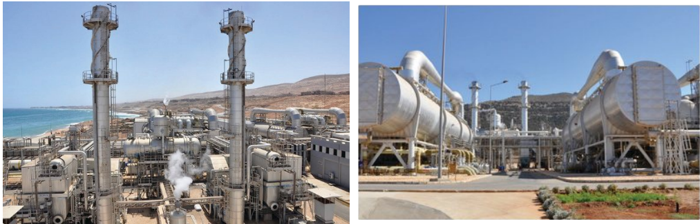
Figure (3). General view of Zuara and Sussa desalination plants each 40,000 m 3 /day.
