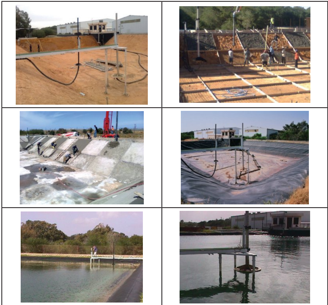
Figure (6). Starting up and maintenance work activities at TESP [3].
